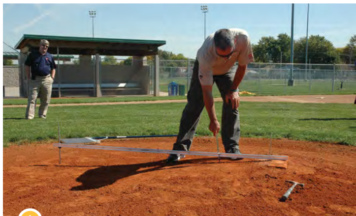
A slope board is a useful tool in maintaining the 1-inch fall per foot mandated for professional, college and most high school baseball mounds.
